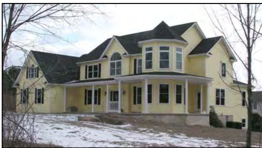
New Home Construction
